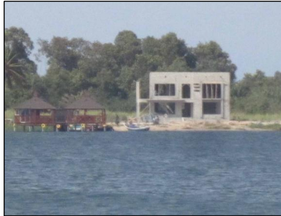
Photo 2.6.4: New, insensitive development is taking place within the Ramsar site at Ada, which, if uncontrolled, will significantly damage the attractiveness of the area for tourism
